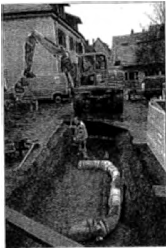
Fig. 5: Installation of an expansion bend in a PE-HD gas pipe, Meiergasse, distance to the well field approx. 80 m in northnortheast direction, March 2009 (Photo: U. Burbaum).
