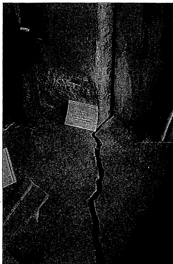
Fig. 3: Tension crack in a baseplate, building Jägergasse, distance to the well field approx. 70 m to the northeast, March 2009 (Photo: U. Burbaum).
